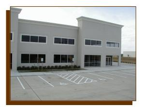
This project consists of two 85,620 SF tilt-wall office/warehouse buildings that were designed to accommodate leases on the southwest side of Houston. The project is designed with flexibility to handle a number of smaller leases or single-building tenants.
